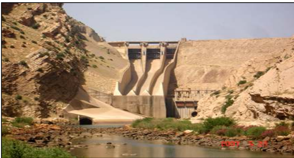
Figure (1): Downstream view of Darbandikhan Dam.
